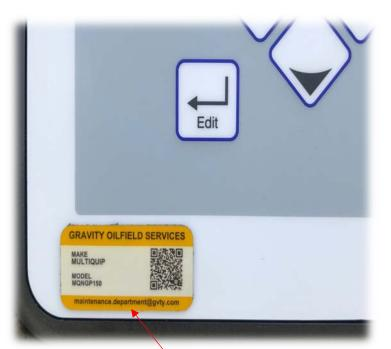
On Natural gas generators equipped with Basler controllers, the QR Code Tag is to be placed on the bottom left-hand corner of the controller.
