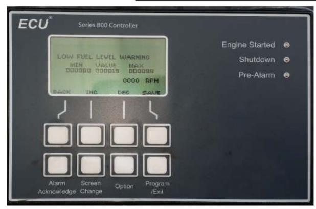
Step 4: Adjust low fuel level warning to desired percentage by pressing the increase or decrease buttons.
