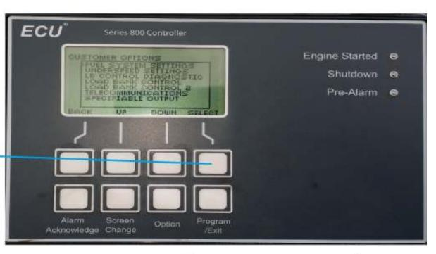
Note: This is a example of how to adjust the low fuel level warning & low fuel level shutdown
